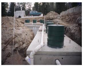
SC3 75000 Complete Treatment System installed with risers and vent pipe. Minimal maintenance.
