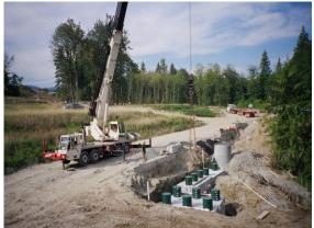
Duplex Pumps, chamber 6000 G, alternation effluent to drain fields. Type 3 expandable tank system.
