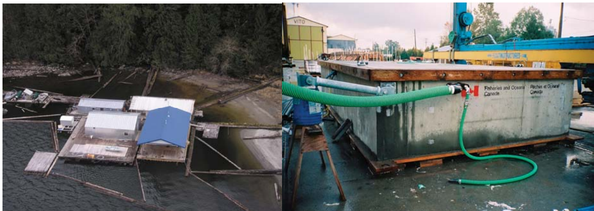
Photo 9 Aerial view of Machmell Federal Fisheries camp and of Go-Green treatment system inside its own float prior to shipping (flexible piping connection shown will be used to connect to float camp plumbing).
